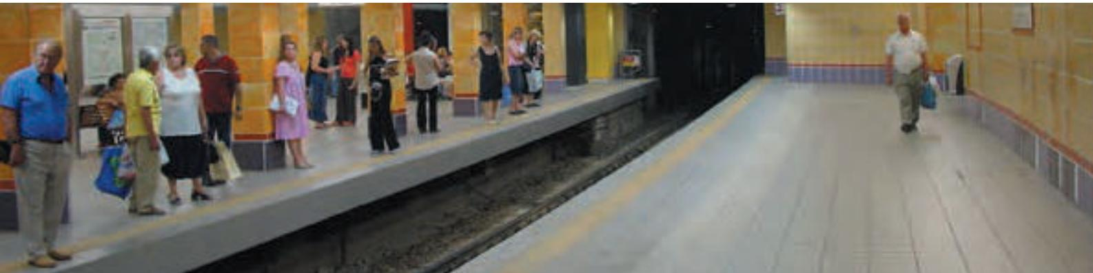
**Granitogres Tactile** is a special language, imprinted on fine porcelain tiles, able to guarantee greater autonomy and safety for the visually disabled when they have to move around. The modular elements in the flooring are arranged in easily understood informative codes, which give directional information and situation warnings through four different channels:
